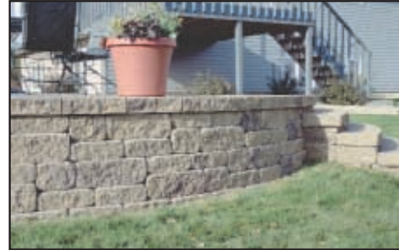
Mosaic retaining walls can feature a variety of design elements like curves, corners, and steps.
